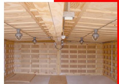
Interior view of clear span duplex magazine
