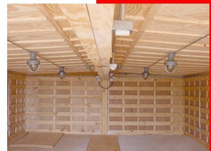
Interior view of clear span duplex magazine
